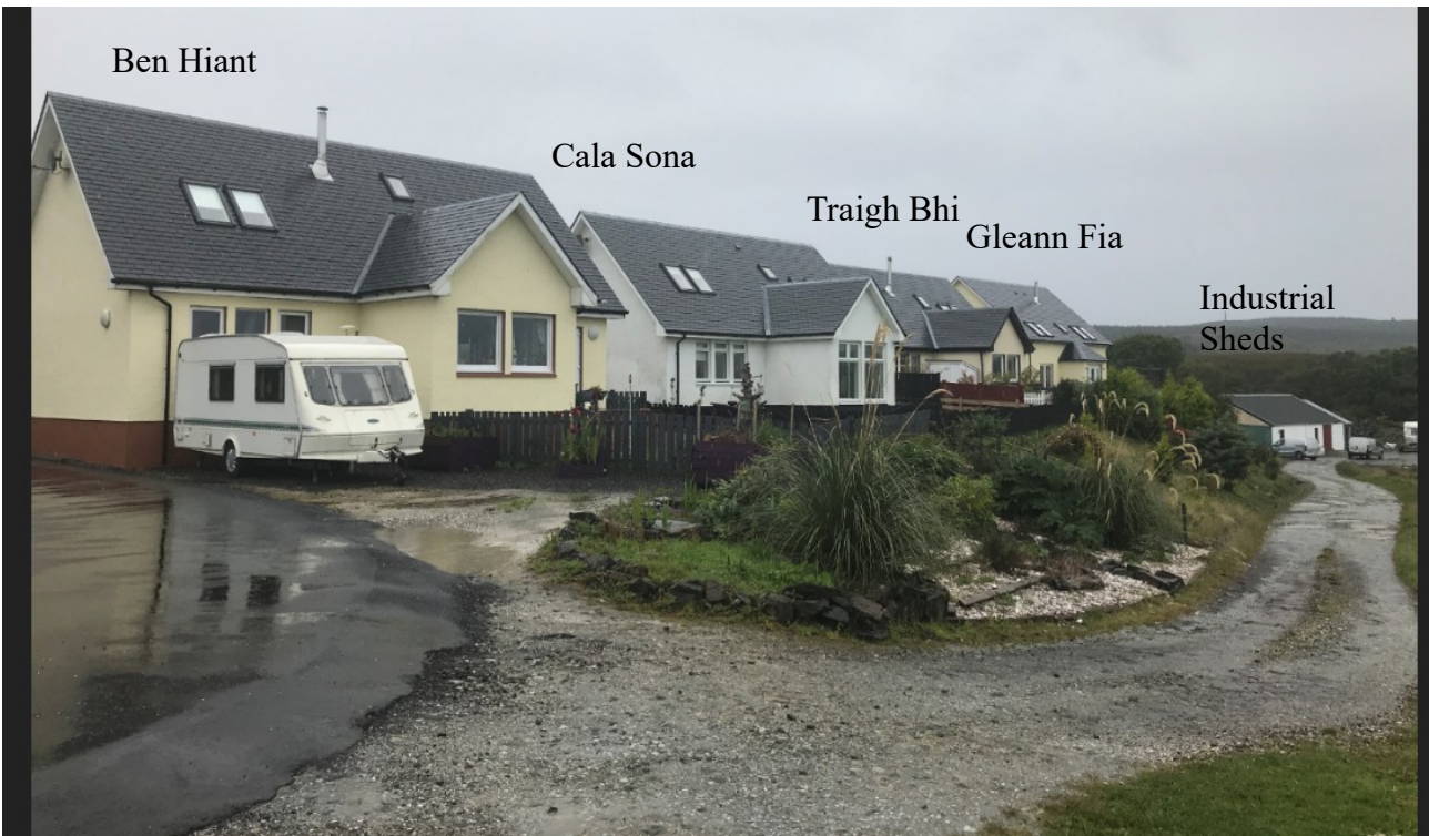
View of all 4 houses from the shared access road (including industrial sheds)
